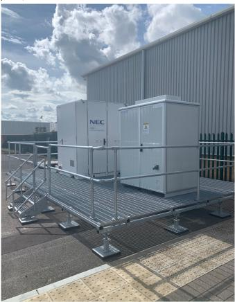
The 280kW/340kWh system from NEC is located in the car park to the rear of the Data Centre and incorporates its own fire suppression system and fully automated controls. The BESS will cycle (charge and discharge) every day to produce the savings and revenue for both EOS and Timico.
